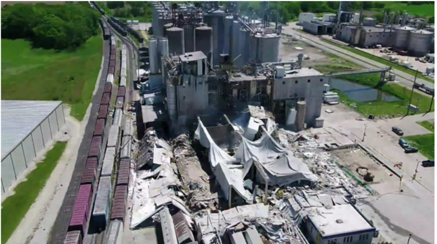
Figure 1: Didion Milling Company's Cambria Wisconsin Facility following May 31, 2017 Dust Explosion 2
