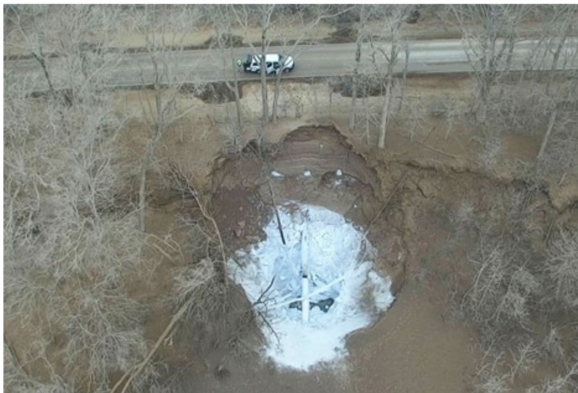
Figure 2: Pipeline Transfer Rupture Effects (Source: EENews.net)
